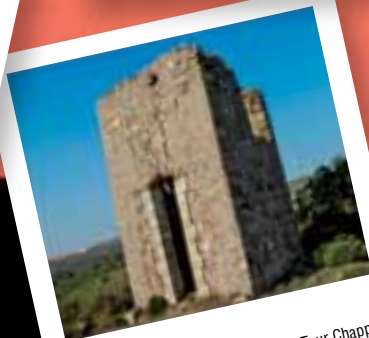
La Tour Chappe
